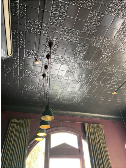
ground floor ceiling
